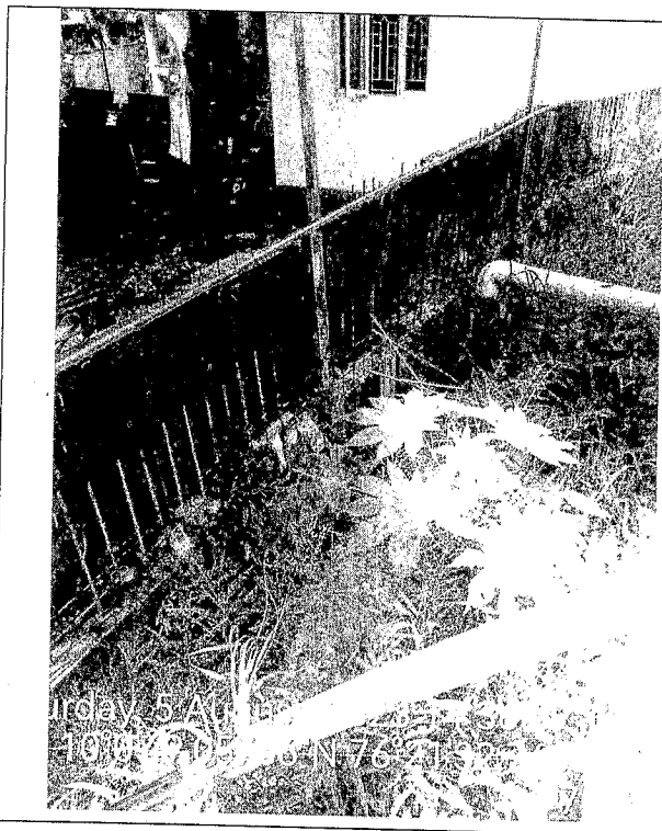
Drainage channel at the boundary of M/s. PHG and Link Valley compounds- See the silted portion of the channel and many inflow pipes provided
