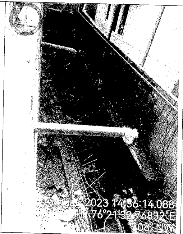
Drainage channel at the boundary of M/s. PHG and Link Valley compounds- See the silted portion of the channel and many inflow pipes provided
